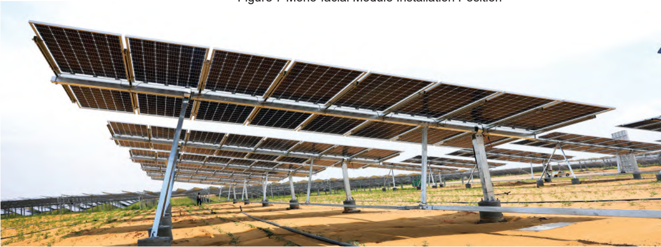
Figure 7 Mono-facial Module Installation Position
